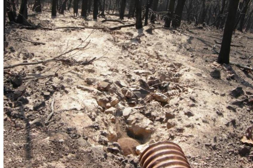
Channelized flow at drains → resulting in high connectivity with streams
