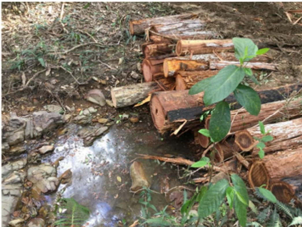
**Figure 4: Temporary log crossing with water in ephemeral stream below crossing, Wauchope region, NSW. Source: NSW Forestry Corporation**
